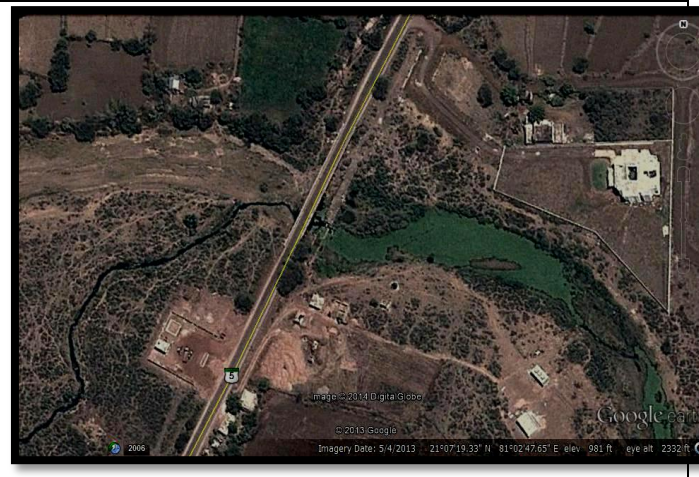
Plate 2. Municipal Sewage Drain In Parrinala North Direction of city
